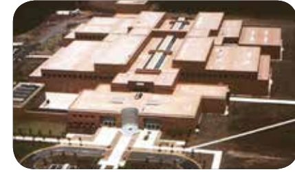
Trident Training Facility Kings Bay, GA
